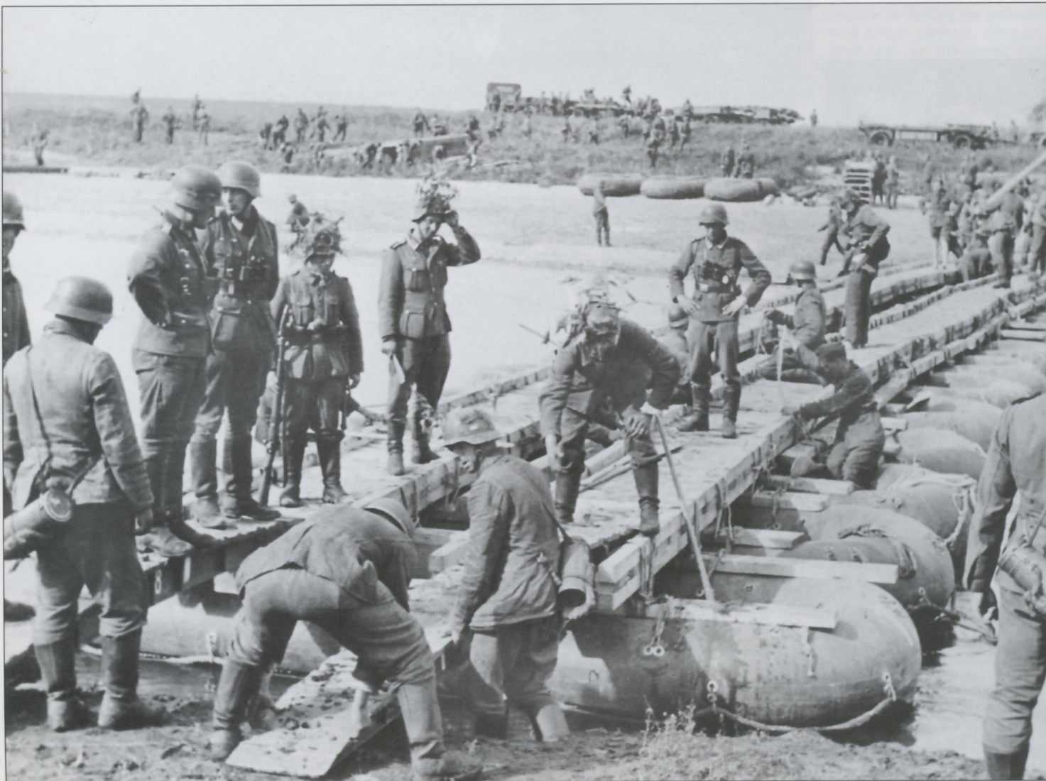
Pioneers are setting a 4-meter aluminium light assault bridge section in place as a ramp to bridge the gap to shore from a recently completed pontoon bridge. Pre-fabricated wooden road-bed sections were laid atop medium inflatable boats to form a pontoon bridge capable of handling trucks and light tanks. A single inflatable boat could support 1.35-tons and had a 6-foot beam with an 18-foot length. On the far shore are the bridging column's trucks and trailers, which were used to transport the boats and road-bed sections. These same boats were also used to construct rafts of different capacities using the same road-bed sections. A 2.25-ton raft consisted of two boats; four made up a 4.5-ton raft, and six made up a 9-ton raft. All types of bridging and river crossing means were essential due to the large number of rivers and streams encountered as the Germans plunged deeper into Russia.
