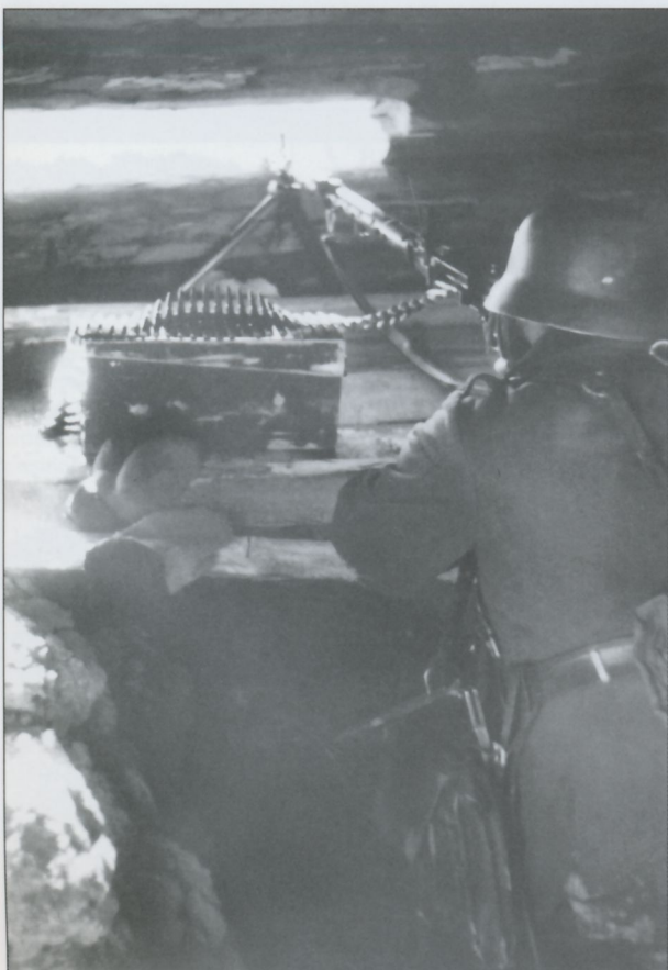
An MG34 machine-gun in action inside a log bunker. The Germans typically constructed wide firing ports in bunkers to allow a broad field of fire, but they kept the height of the opening narrow to make it more difficult to detect and hit with return fire.
