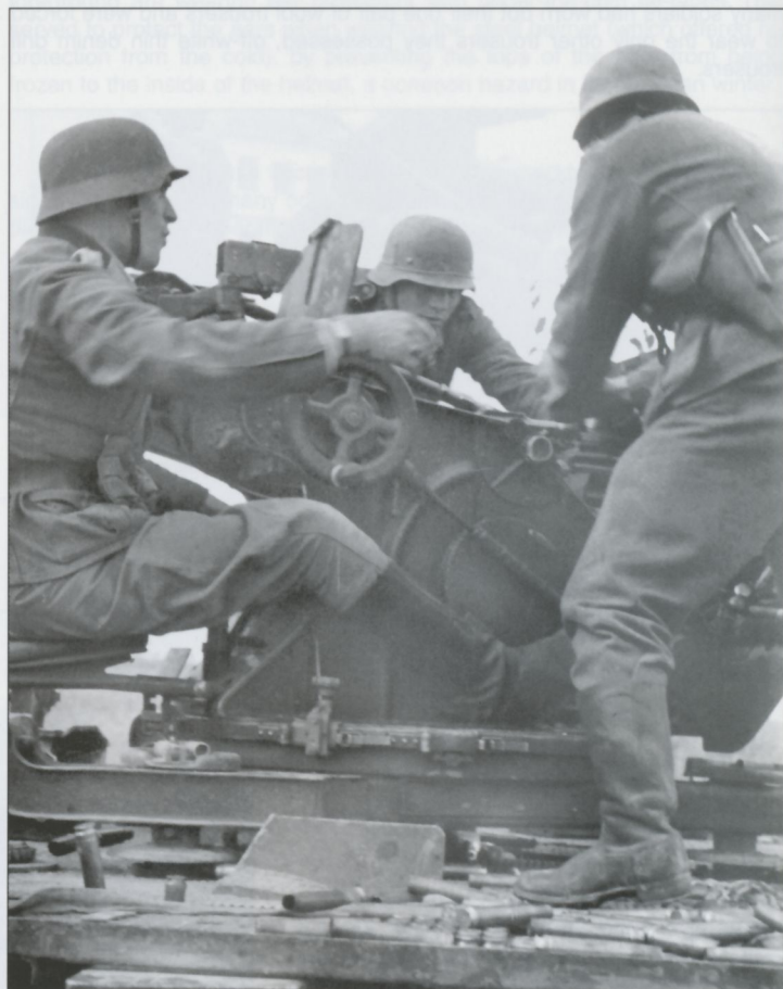
The crew of a 2cm FlaK30 light anti-aircraft gun engages low flying aircraft. This gun, largely replaced by the 2cm FlaK38, remained in use throughout the war. 2cm light FlaK was mainly intended to protect troop formations from air attack and provide close-in air defense of heavy anti-aircraft guns. They were provided both high explosive and armor-piercing ammunition making them suitable for anti-personnel suppressive fire work as well for engaging lightly armored vehicles. As troop strength dwindled, causing depleted infantry units to defend wider frontages, 2cm guns were often assigned to them as effective antipersonnel weapons to break up massed Russian assaults. With a cyclic rate of fire of 280 rounds per minute, these guns were highly valued in this role.
