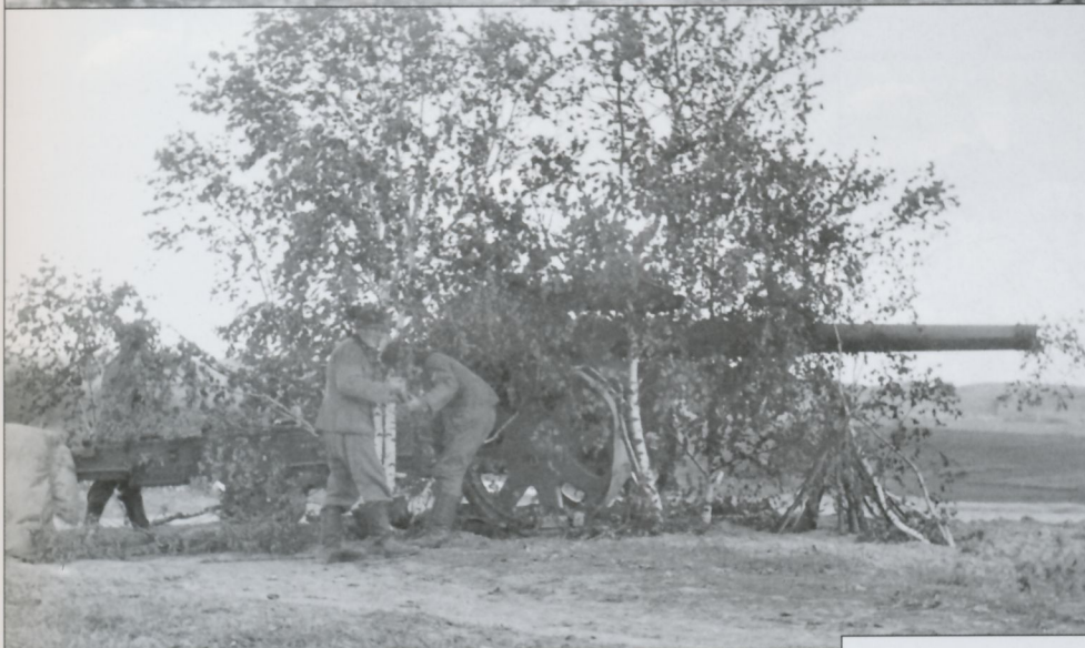
This 15cm s.FH18 heavy field howitzer has been positioned among a few saplings and provided with additional camouflage. The crew's carbines can be seen stacked beneath tree limbs forward of the howitzer. This piece is fitted with aluminium wheels for towing by draft horses. Howitzers intended for motorized towing were fitted with solid rubber tires. This piece remained the principal divisional heavy field howitzer throughout the war. Its maximum effective range was 14,570 yards.
